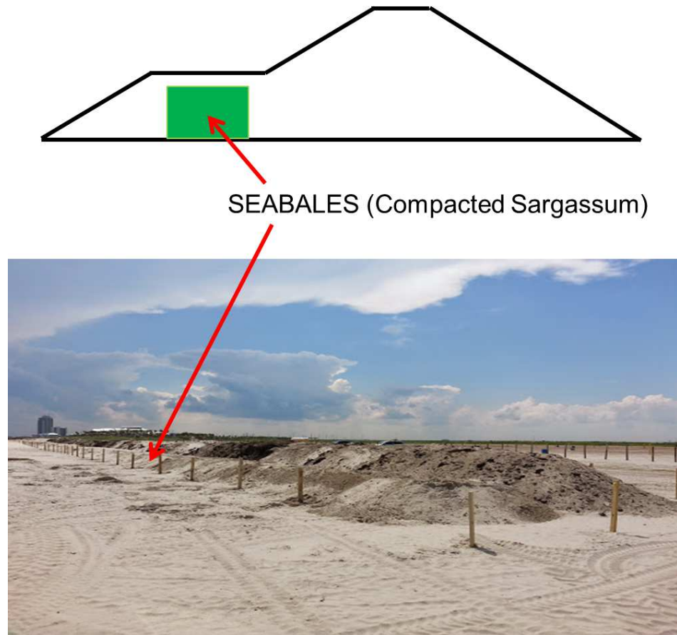
Figure 1.2: Schematic cross-section and prototype photo of seaweed-enhanced dune. Compacted Sargassum bales (seabales) are placed inside the berm of the newly constructed sand dune.
