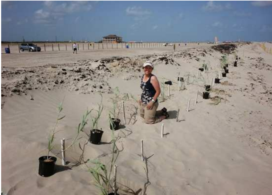
Figure 2.7: Photo of initial vegetation planting. Panicum amarum was planted on the berm of dune segments 1 and 2 after initial dune construction was completed.
