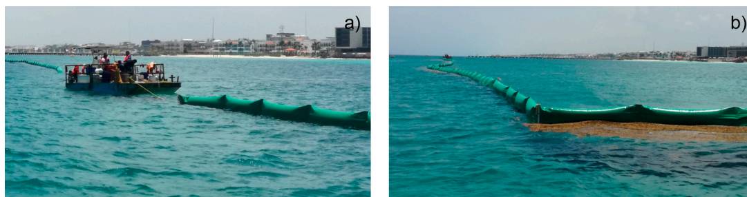
Figure 13. U-shaped barriers to contain sargasso off in Playa del Carmen. (a) Frontal view, (b) lateral view.
